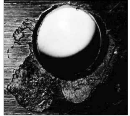
Figure 2. The overlay material in the vicinity of one of the oil holes. Note the well defined edges where the overlay material has lifted.
