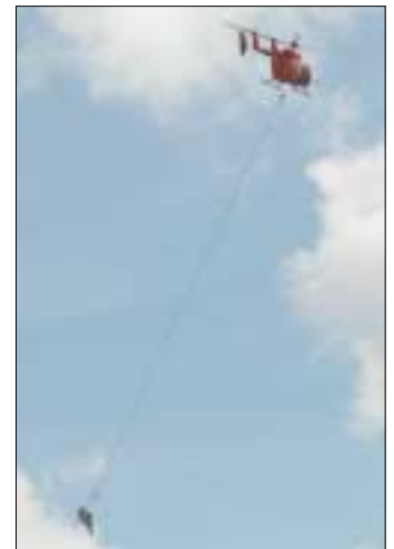
Linesmen suspended 100 feet below the helicopter!
