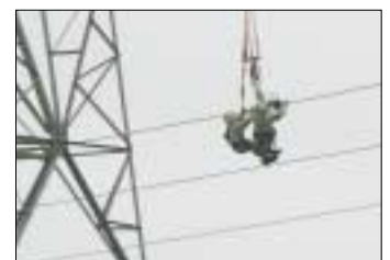
Linesman wearing special suits are able to handle live conductors at 220,000 Volts!
