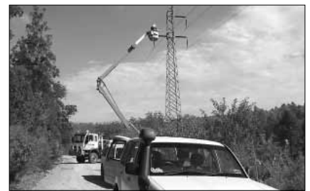
Using an EWP to place the OHLCD on a conductor.
