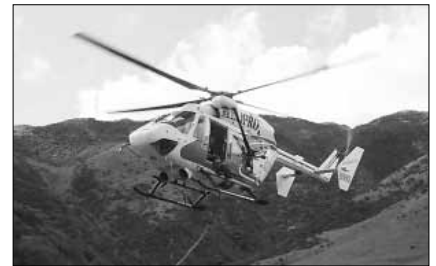
Using a helicopter to put the OHLCD on a conductor.
